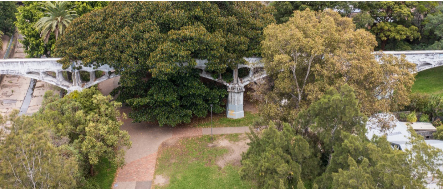
↑ First reinforced concrete structure in Australia: Johnstons Creek Sewer Aqueduct, built in 1895 (Annandale, NSW 2021)
