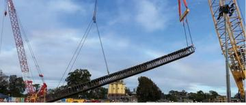
D-wall cages supplied with inclo pipes and earthing sleeves and bridges, which meant the complete system did not require any further work once delivered to site.
